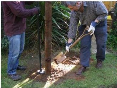
**3. Fill in the hole with the soil taken out and compact regularly**
