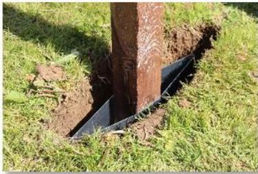
**2. Dig a 'T-shaped' hole, put the fence post with FenceFins™ in**
